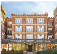
3 Hampton Court 1223 Beacon Street
