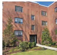
5 Longwood Green 98-114 Sewall Ave
